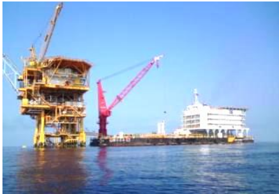
Accom. Work Barge POS1 (300Pax)
