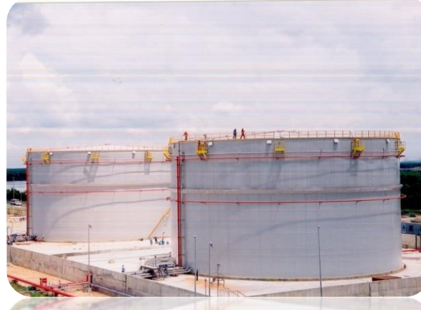
NCS Condensate Storage Project
